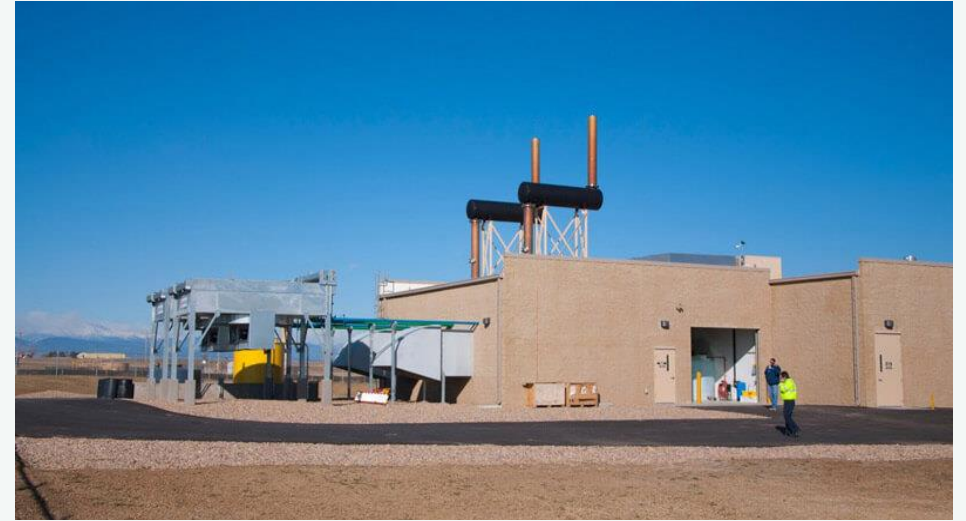
Archaea Energy's landfill gas to energy plant
